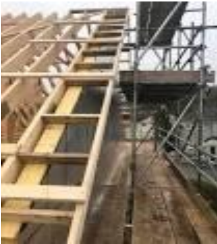
Figure 16 Roof ladder construction
