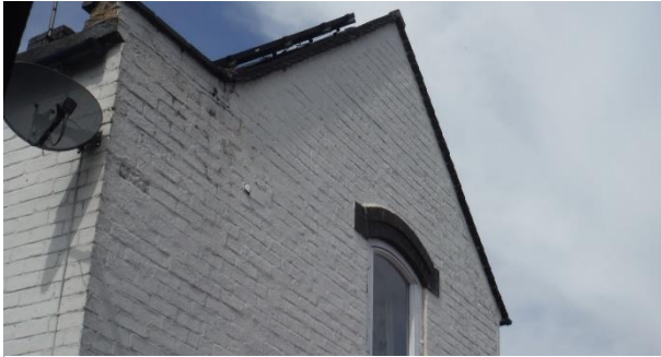
Figure 18 Gable end with flat parapet roof section
